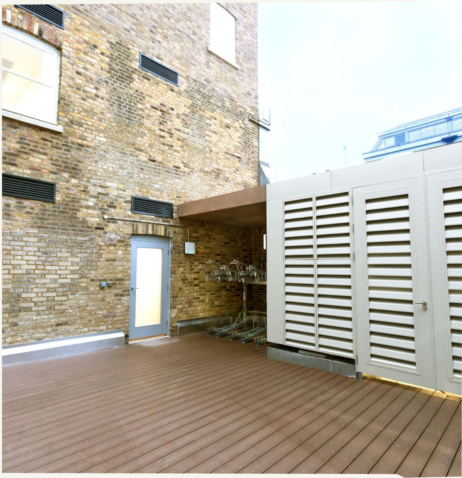
Terrace and bike storage
